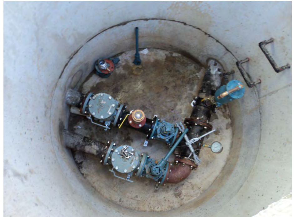
Submersible lift station with valve vault (courtesy of Bemidji Area IHS)
